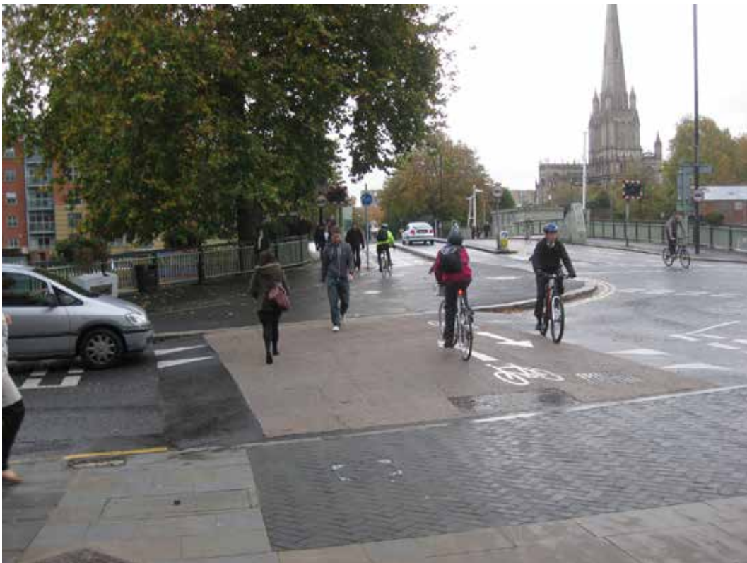
Photo 6.11 – Priority crossing of cycle track over side road, Bristol
