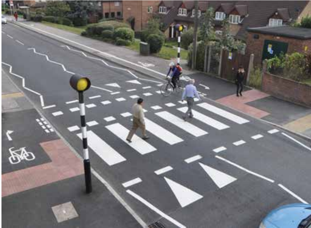
Photo 6.21 – Parallel Crossing for Pedestrians and Cyclists (installation in advance of revised TSRGD)
