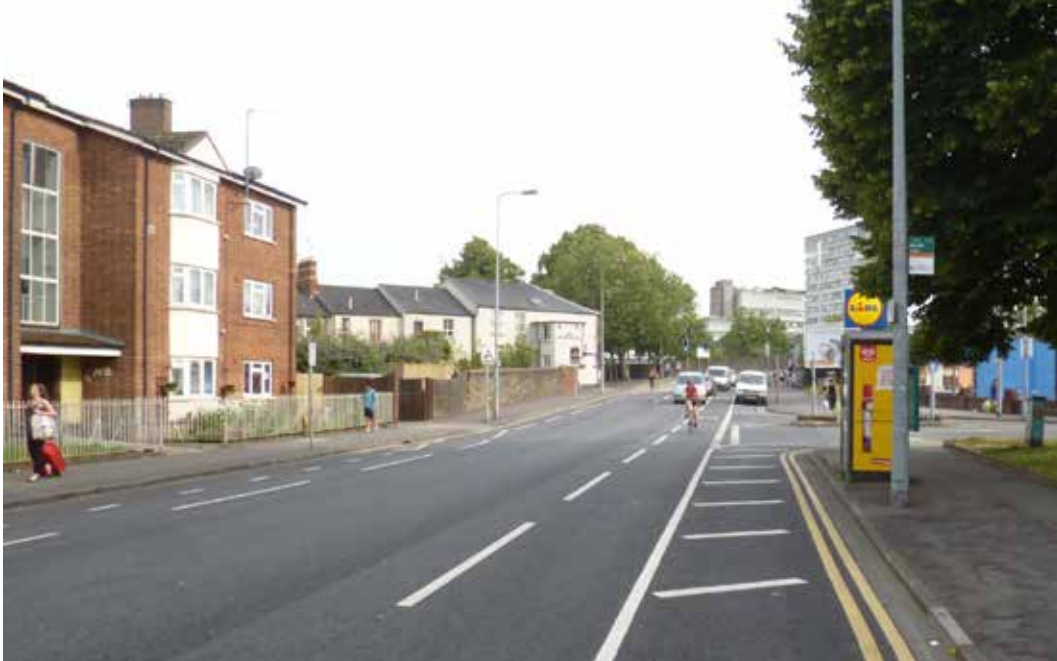
Photo 6.7 Cathays Terrace, Cardiff – Centreline removed to allow advisory cycle lanes to be introduced
