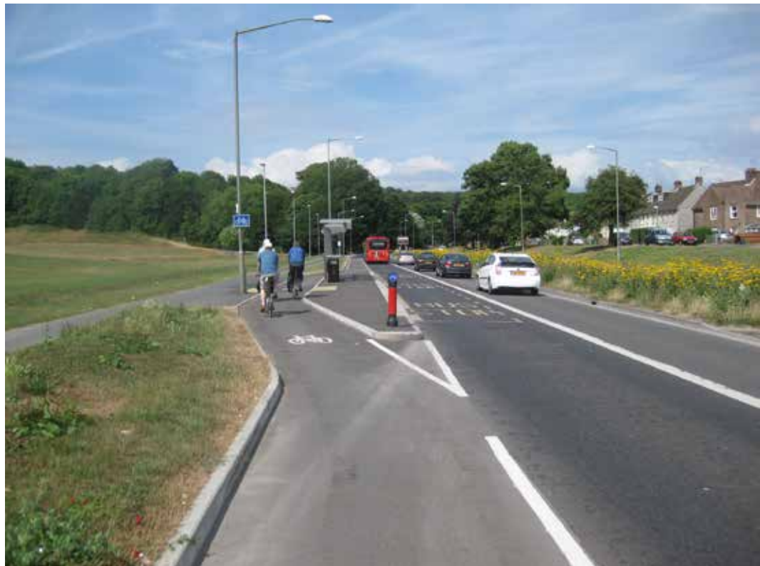
Photo 6.14 – Bus Stop Bypass, Brighton
