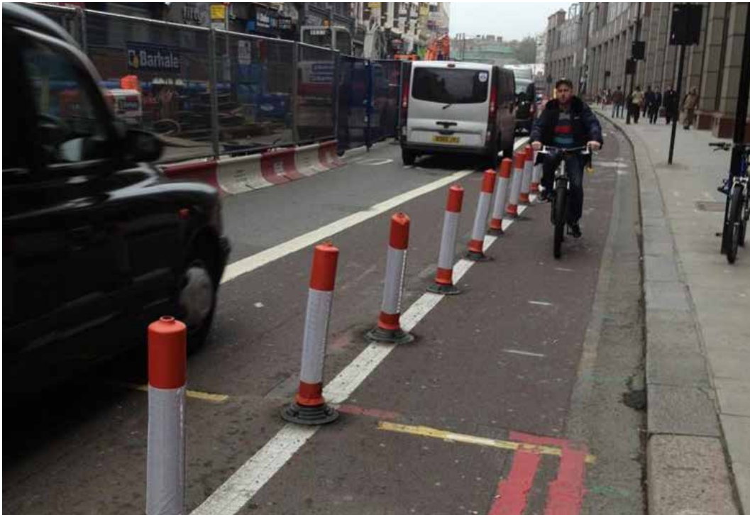
Photo 10.2 – Temporary contraflow cycle lane during roadworks, London
