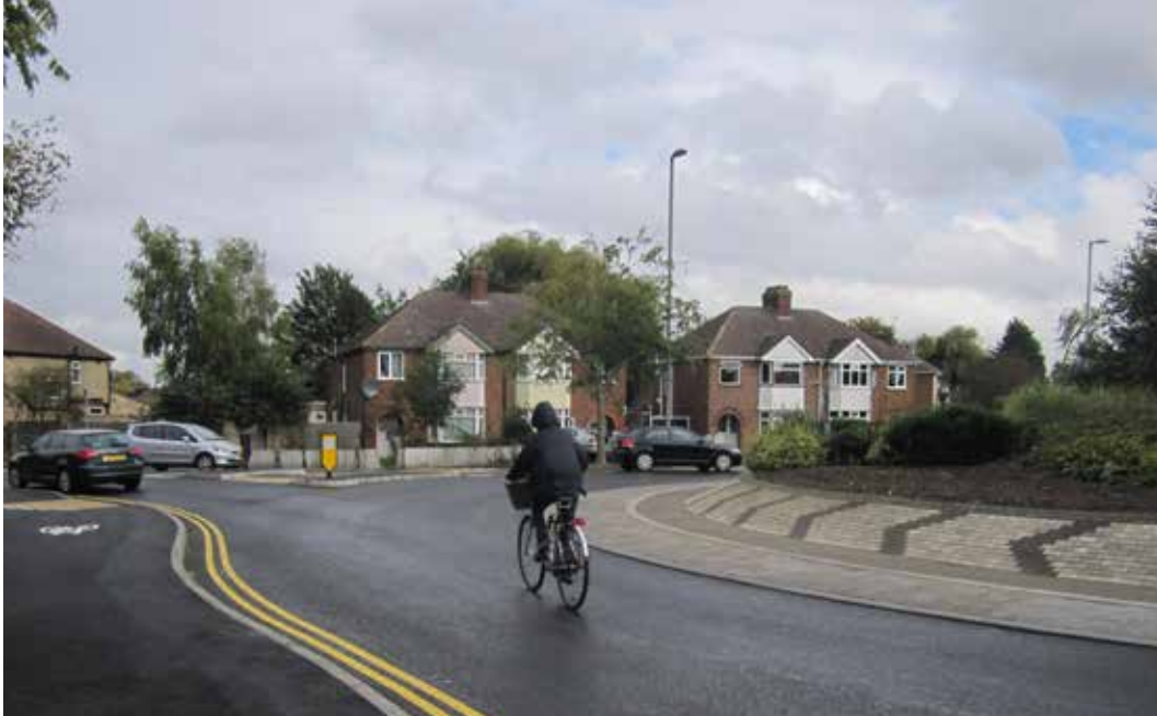
Photograph 6.39 - Compact roundabout, Cambridge, as built
