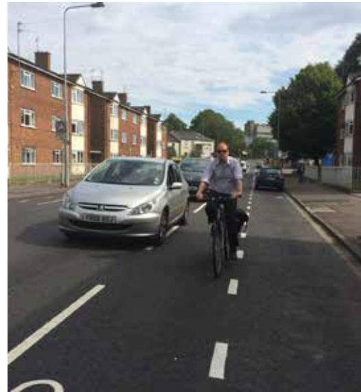
Photo 9.1 a/b/c – Cycle lanes were widened to 1.8m on Cathays Terrace, Cardiff, during resurfacing
