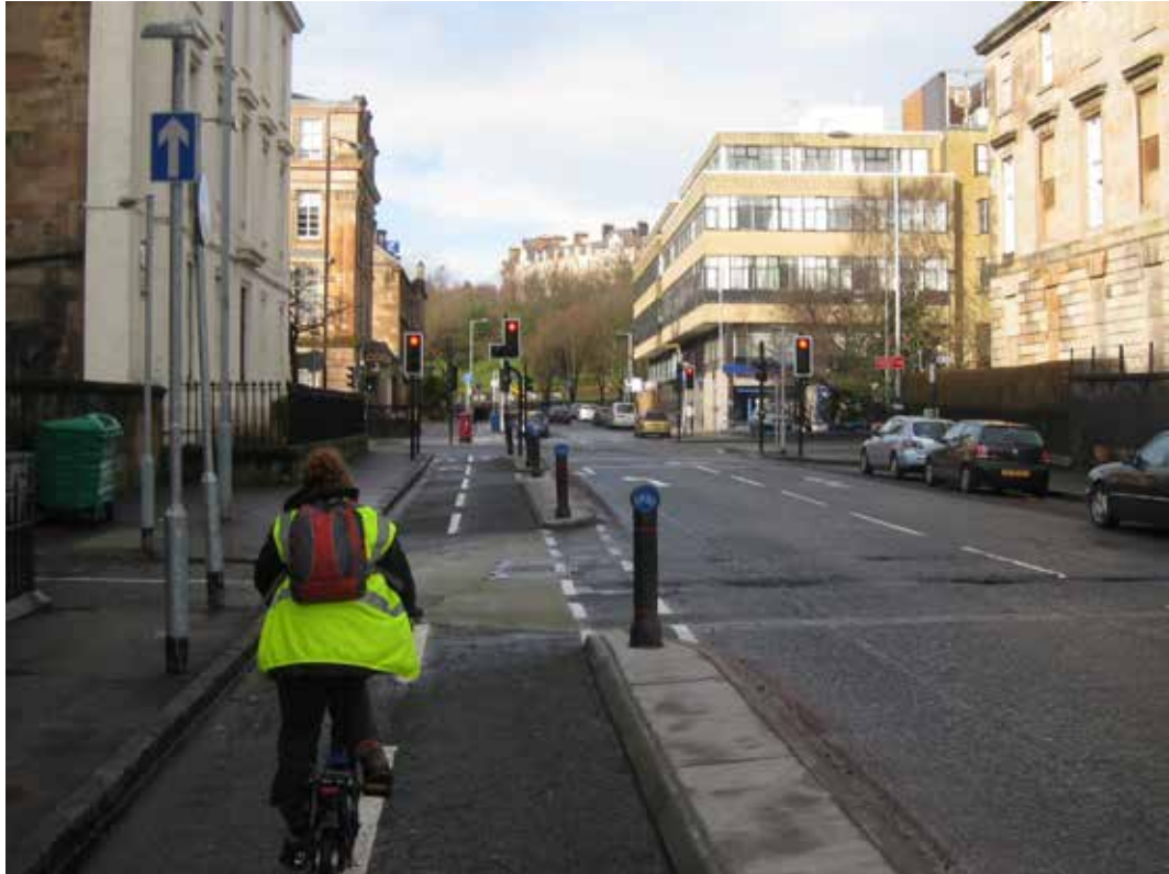
Photo 6.1 - Reallocating carriageway space to cycling enabled this two-way segregated track to be created in Glasgow
