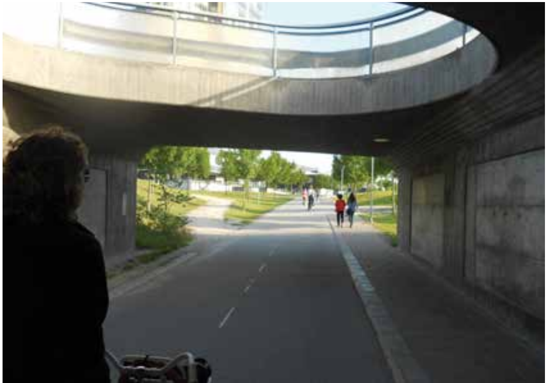
Photo 6.24 – Segregated pedestrian/cycle route beneath busy intersection with good natural light – Lund, Sweden
