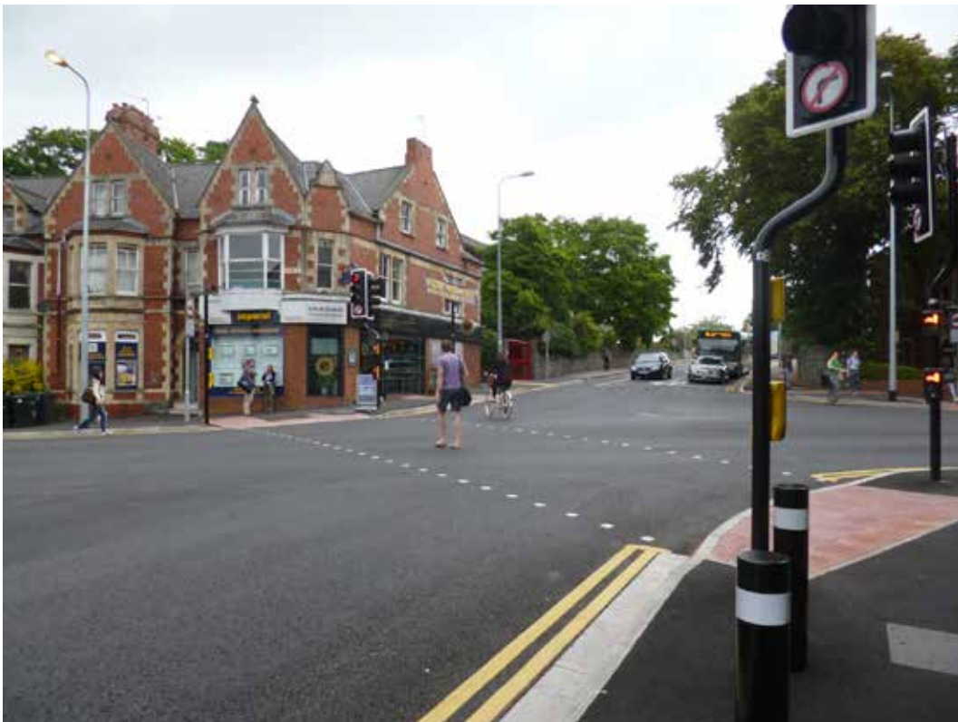
Photo 6.30 – Signalised Diagonal Cycle Crossing, Cardiff
