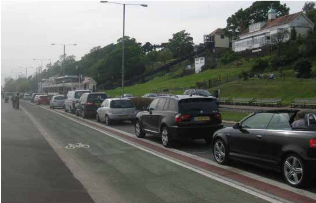
Photo 6.3 – Segregated footway and cycle track at Southend, using contrasting colour and a flush kerb to separate pedestrians and cyclists
