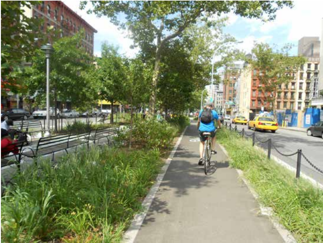
Photo 6.13 - One way cycle track in central reservation, New York City
