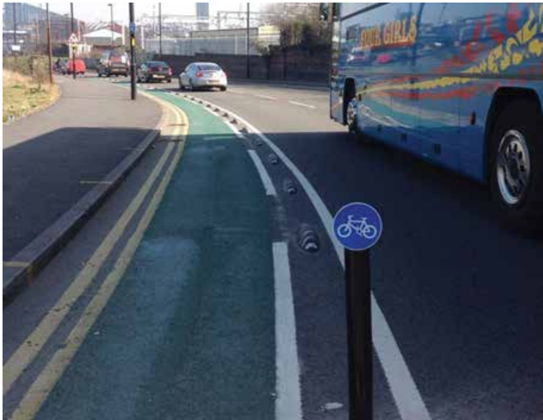
Photo 6.9 – Light segregated cycle track with wand at start, Salford, Greater Manchester (Note – only one lane marking, outside the raised features, should be used).
