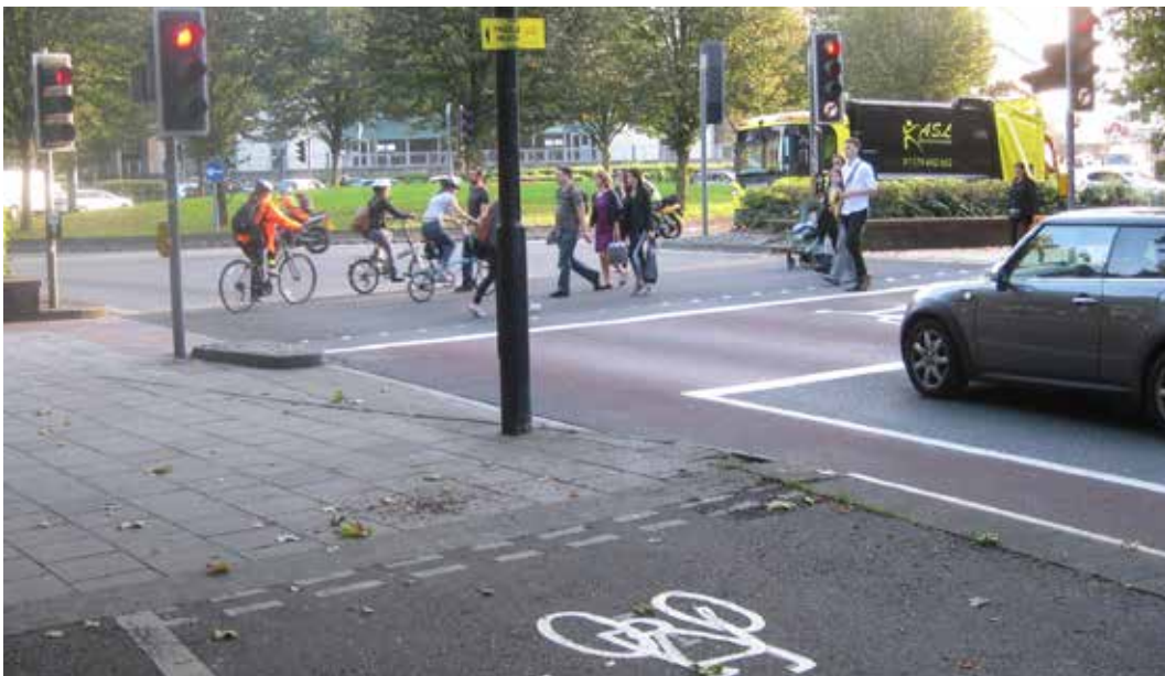
Photo 6.37 – Signalised Roundabout at Temple Quay, Bristol, with cycle facilities on carriageway and separate cycle track around the junction.
